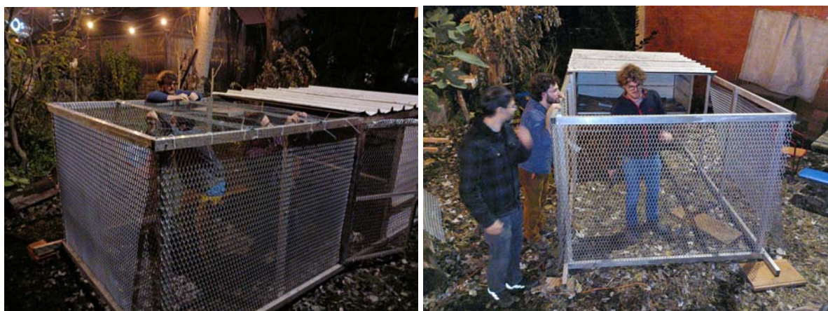
Fig. 14 Replacing the old metal wire with new steel fences to better protect the hens against any predator.
