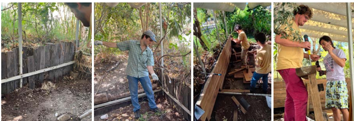
Fig. 11 Construction process of the new bench at the C2 shelter.
